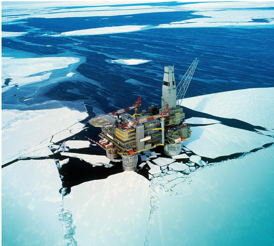
**Figure 3: Sakhalin II platform with multi-shaft GBS in level ice. (Photo: Sakhalin 2)**
