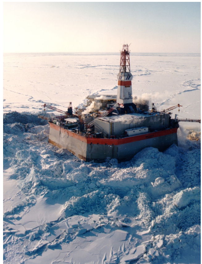
Figure 1-21. The Molikpaq Caisson
