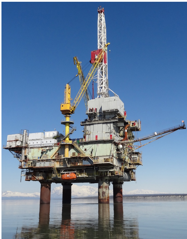
Figure 1-29. Cook Inlet Platform with Tower Type Jackets
