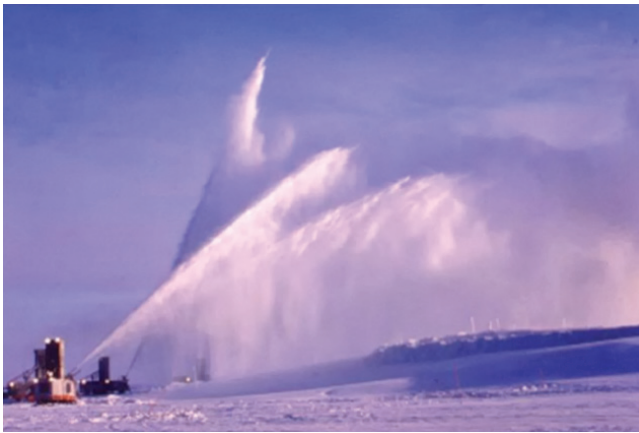
Figure 1-31. Spray Ice Island Construction
