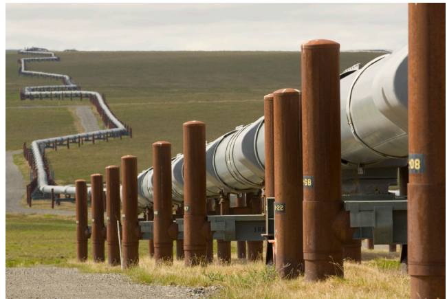
Figure 1-26. Trans-Alaska Pipeline Zigzag Design
